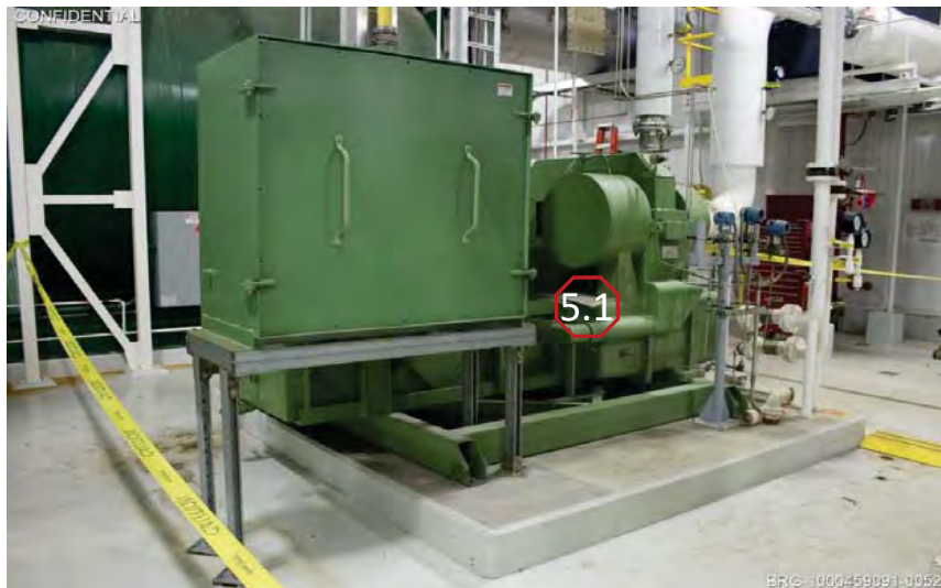
Picture 100045909-14 - Compressed Air System
