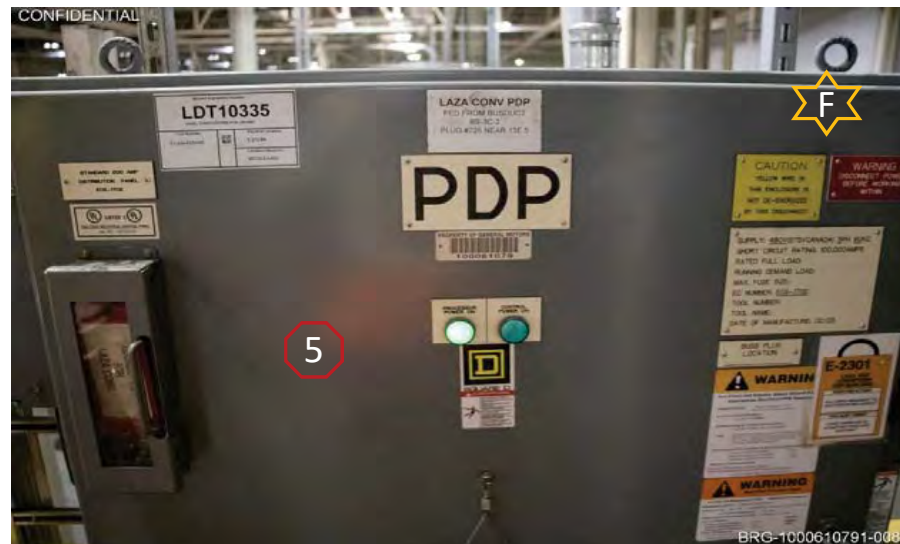
Picture 100061079-12 - Power Distribution Panel
