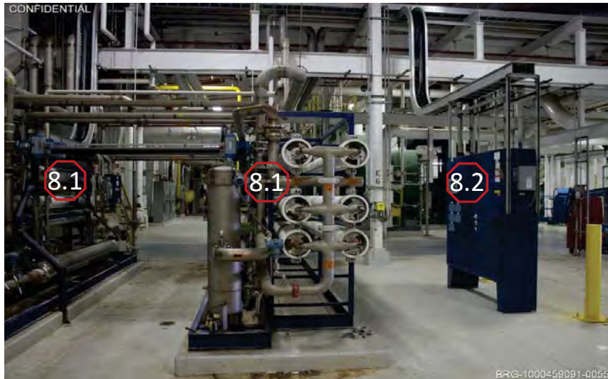
Picture 100045909-23 - Water Treatment System
