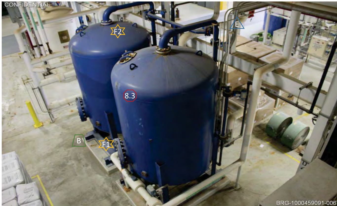
Picture 100045909-27 - Water Treatment System (Water Softening System)
