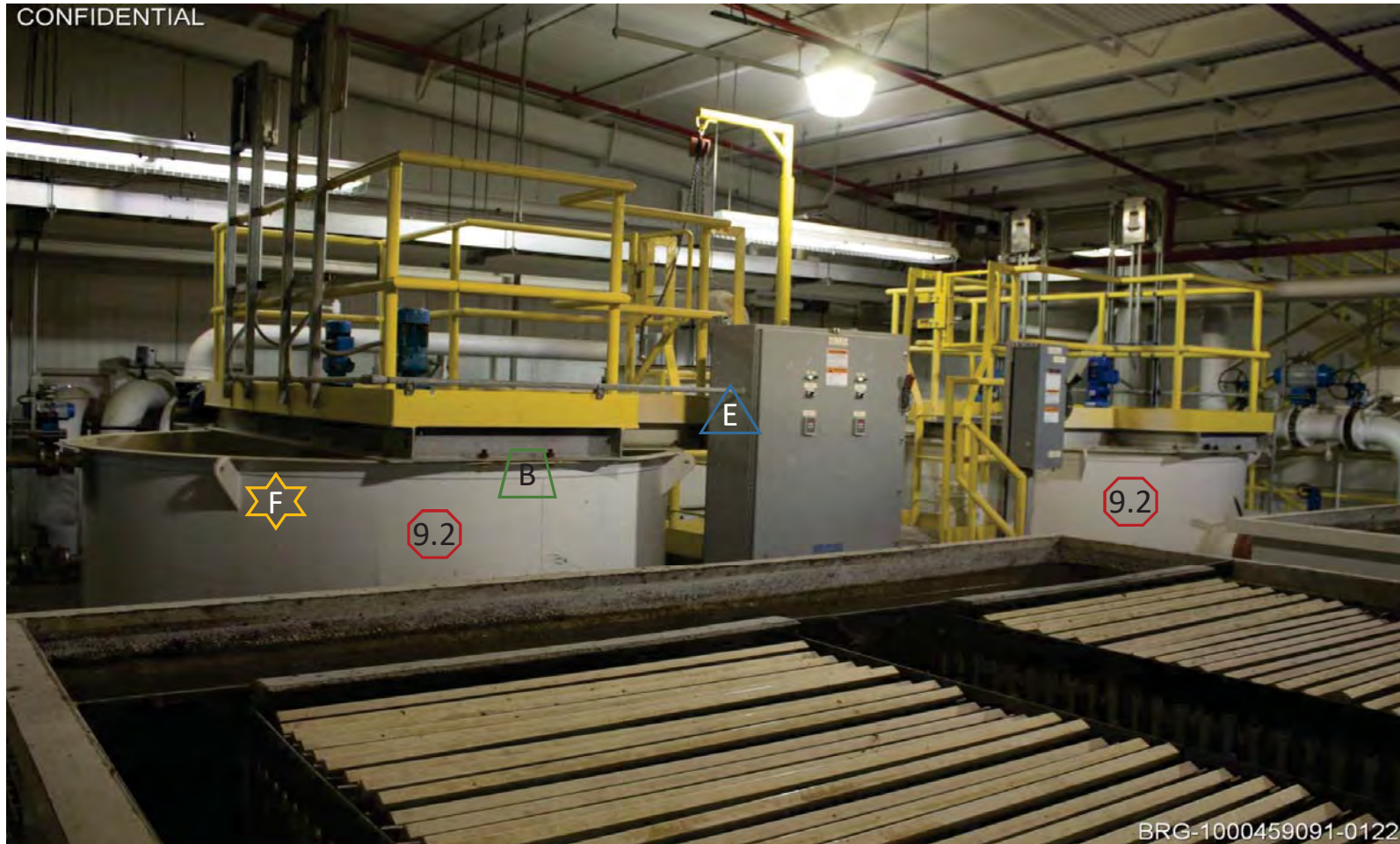
Picture 100045909-33 - WWT (Flocculation Tanks)
