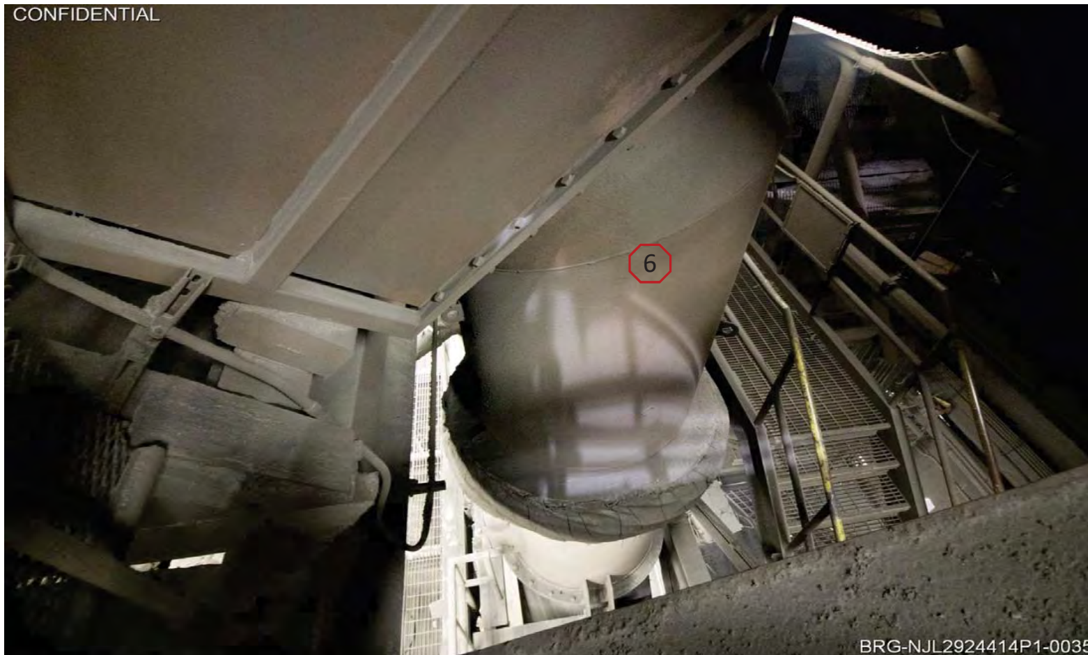
Picture NJL2924414P-3 - Cupola Gas Take-off Duct
