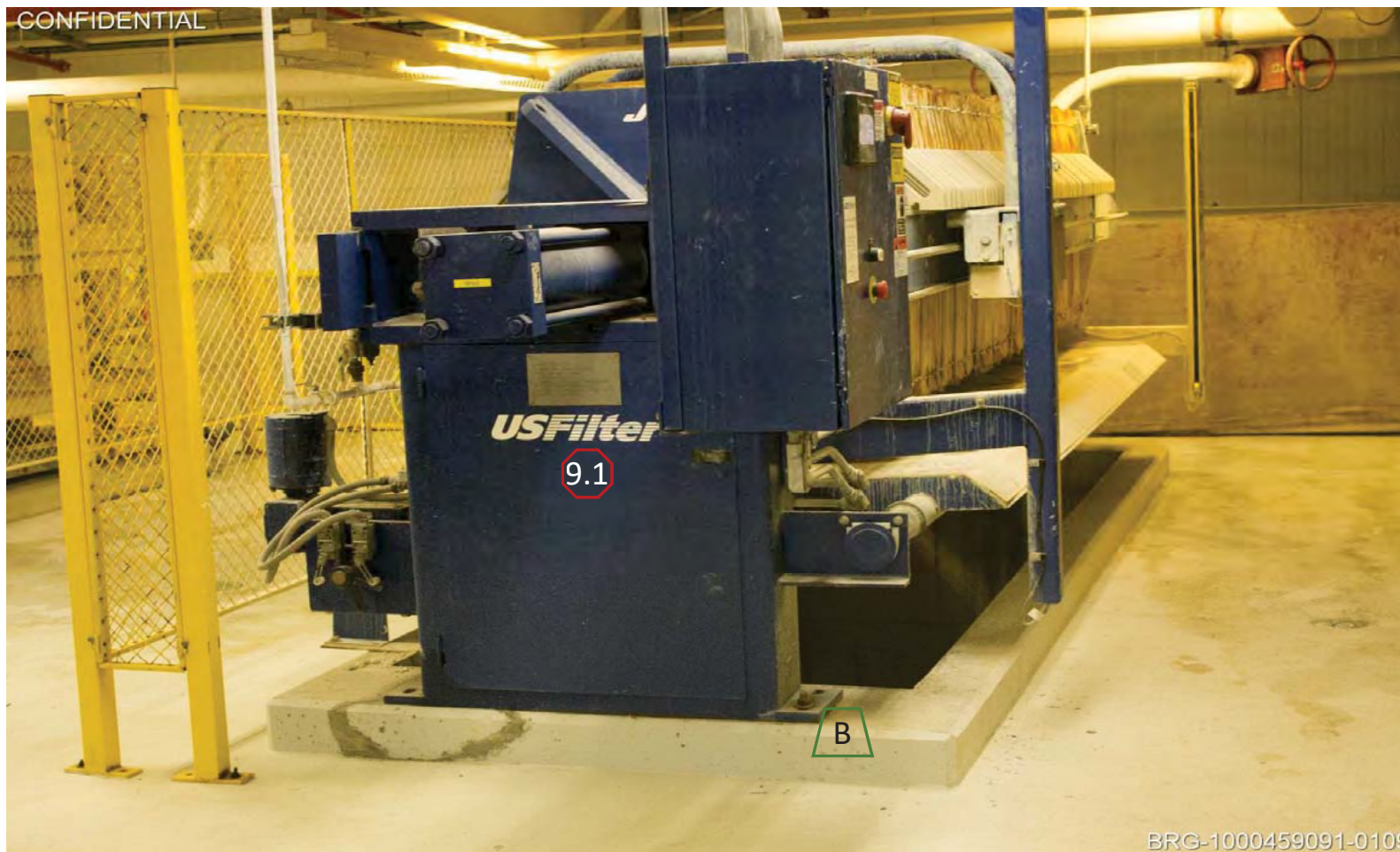
Picture 100045909-32 - WWT (Filter Presses)
