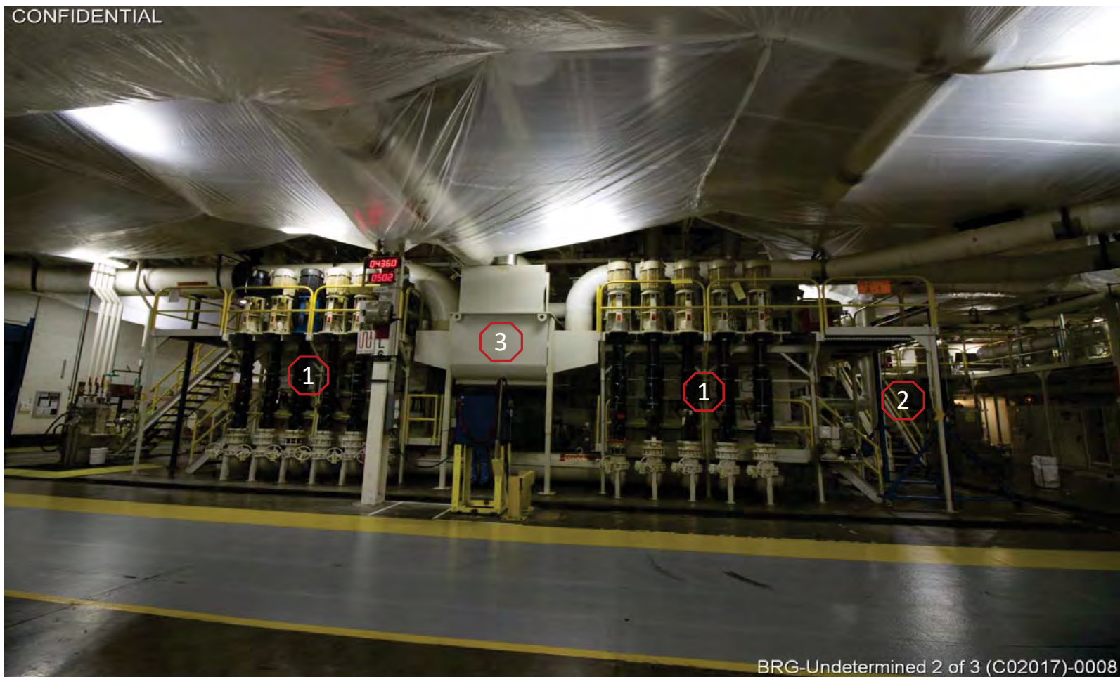
Picture 100070012-2 - Coolant Filtration System
