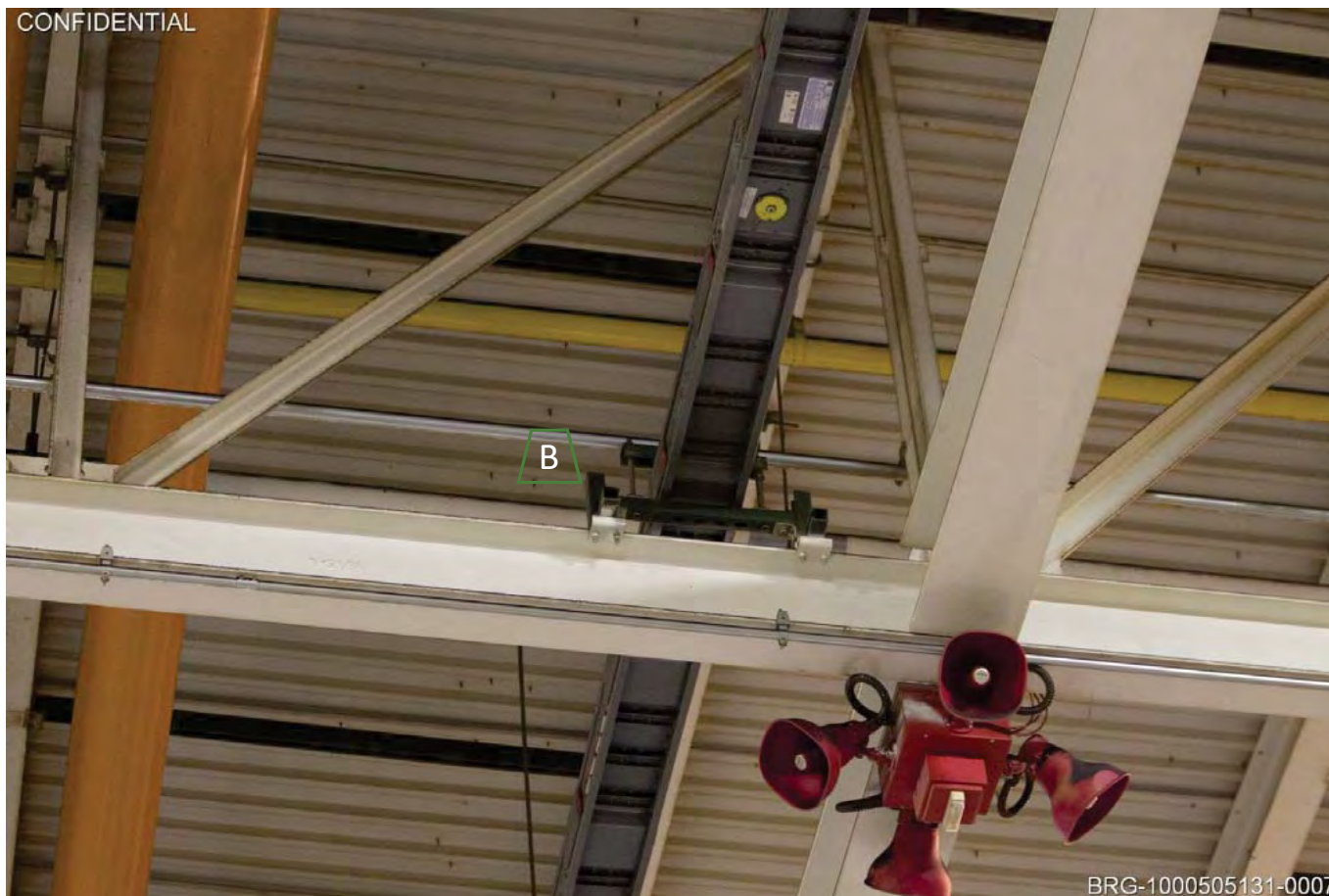
Picture 100050513-2 - Weld Bus Duct
