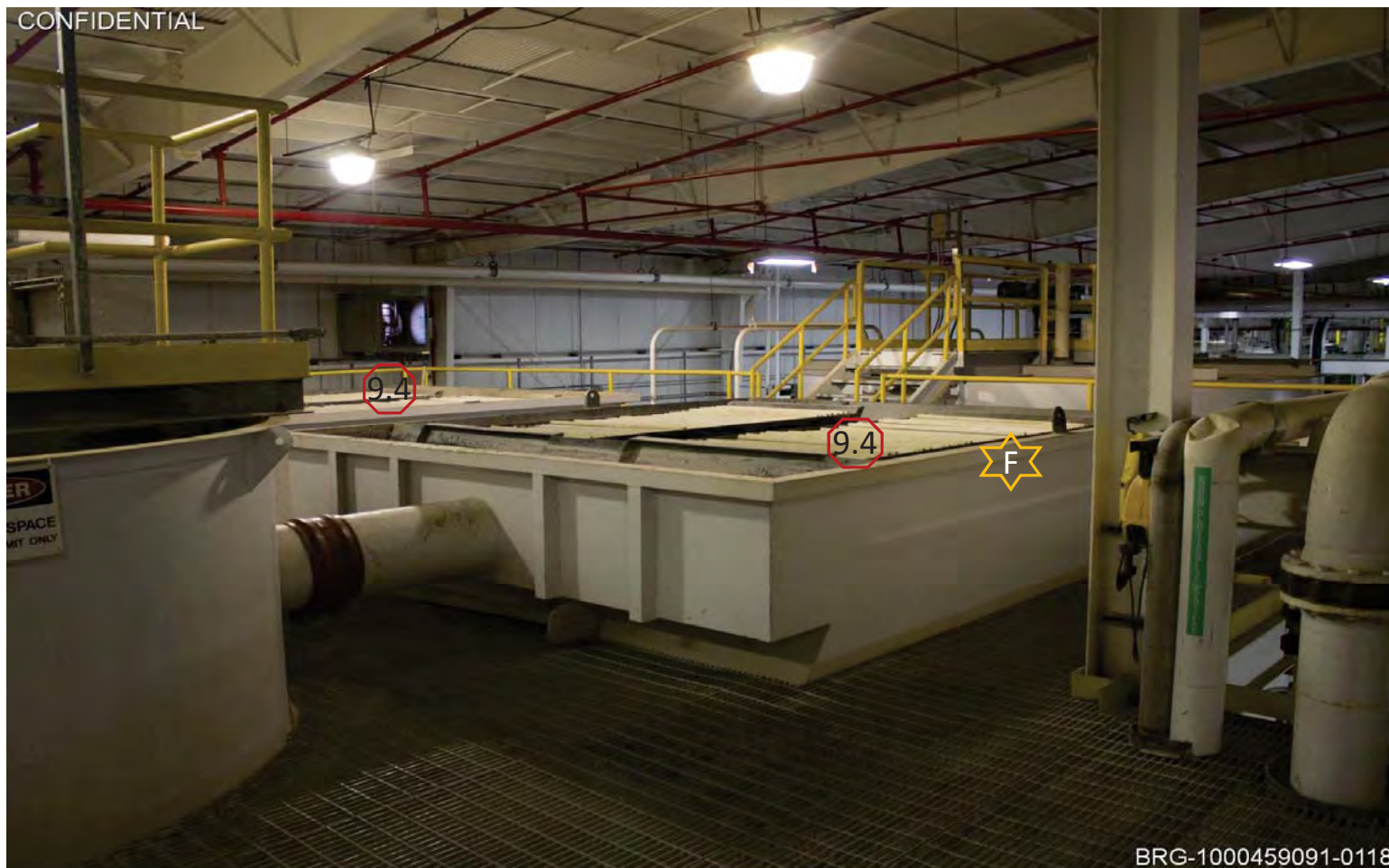
Picture 100045909-37 - WWT (Parallel Plate Clarifiers)
