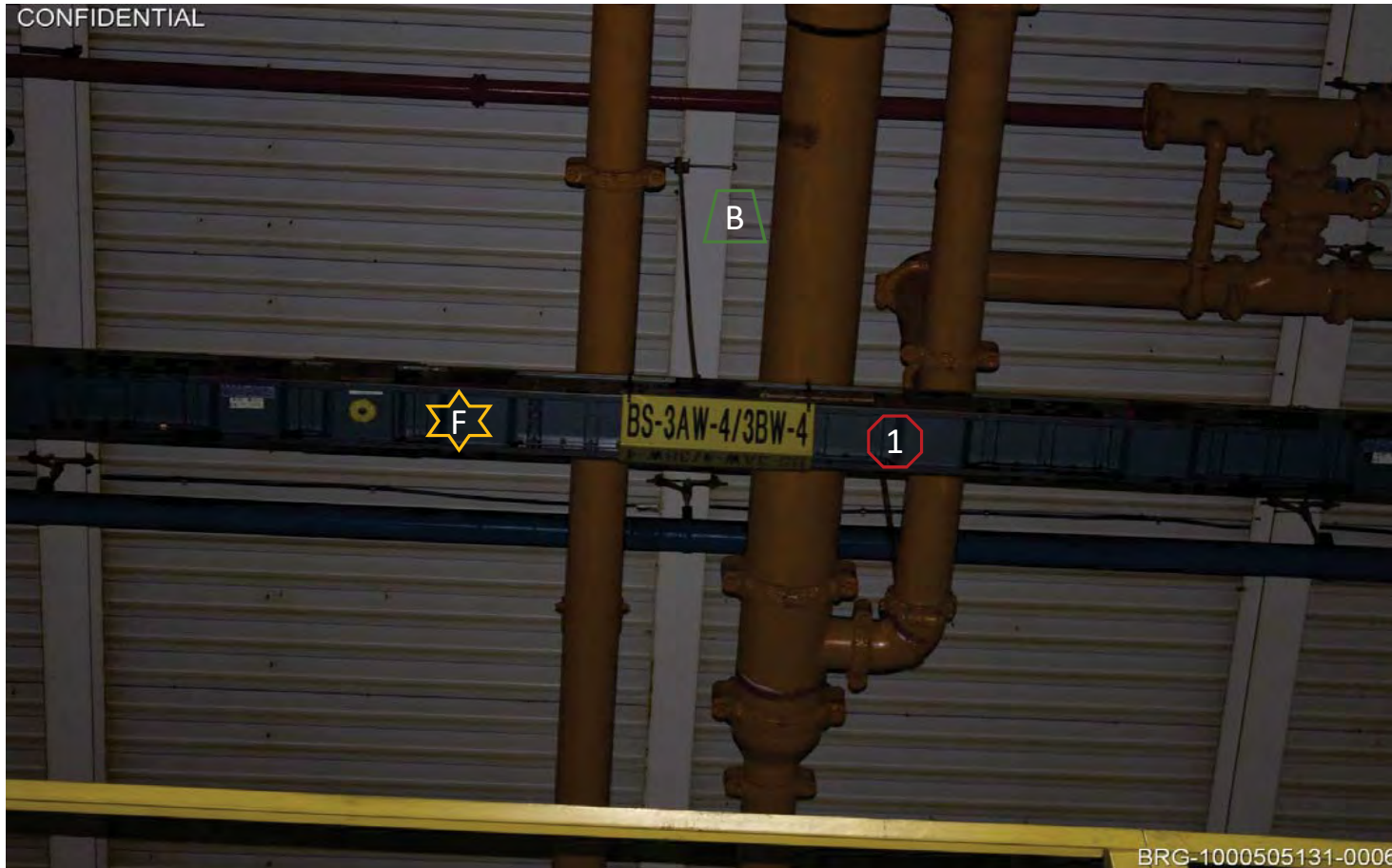
Picture 100050513-1 - Weld Bus Duct
