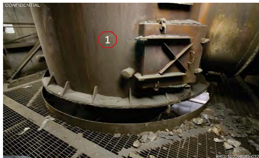
Picture 100098085-3 - Thermal Oxidizer Bottom Section
