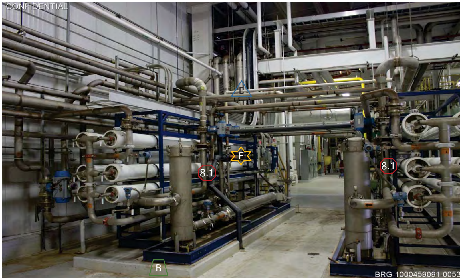
Picture 100045909-26 - Water Treatment System (Reverse Osmosis Units)
