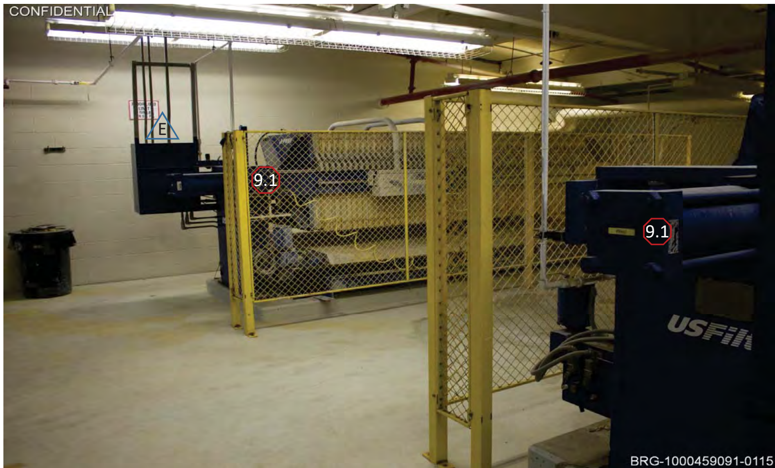
Picture 100045909-31 - Wastewater Treatment "WWT" (Filter Presses)
